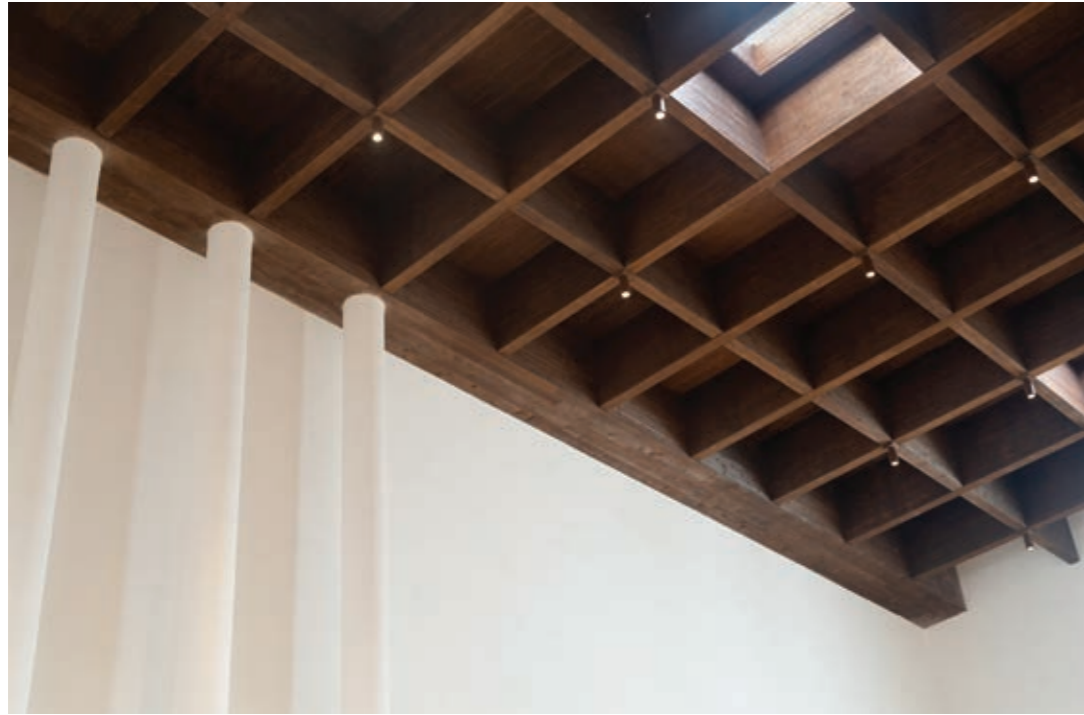
To illuminate the central hall, cylindrical luminaires are mounted on the ceiling at intersection between the wooden beams.
