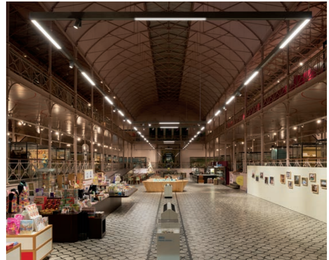
Suspended rectangular luminaires with direct/indirect RGB colour-changing technology characterises the new lighting scheme of the Victoria & Albert Museum of Childhood.
