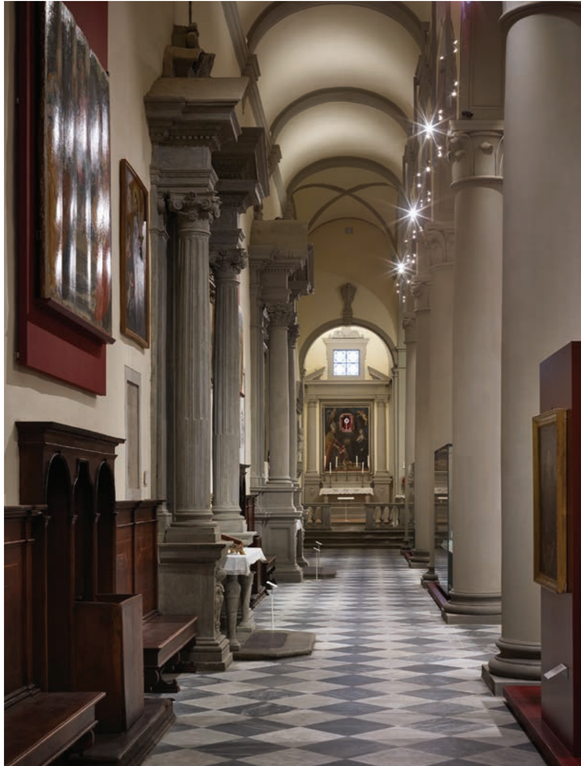
The linear suspension rods, made specifically for the project, are positioned between the columns that separate the central from the side naves.
