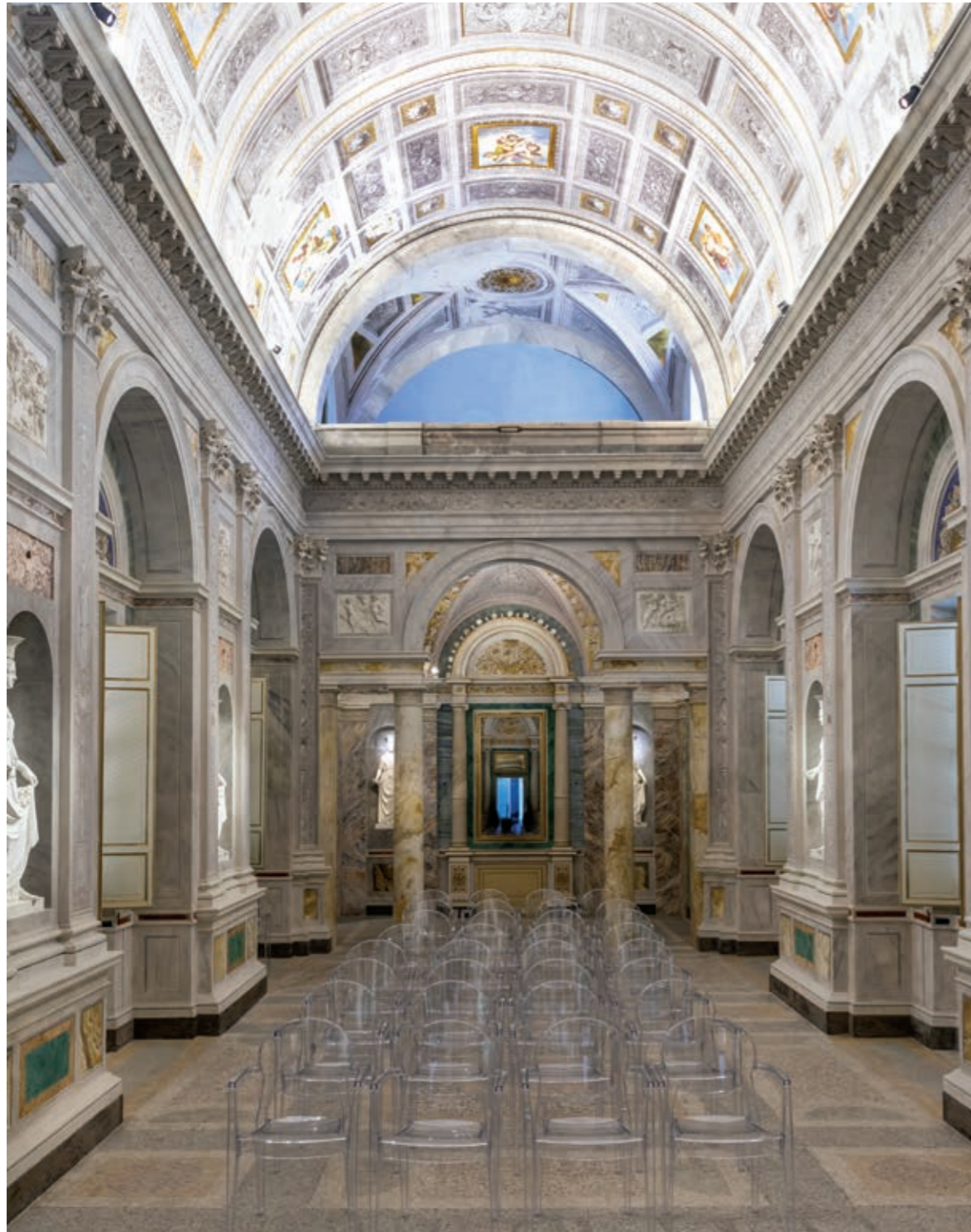
The lighting of the barrel vault uses modular linear luminaires positioned on the cornices.
