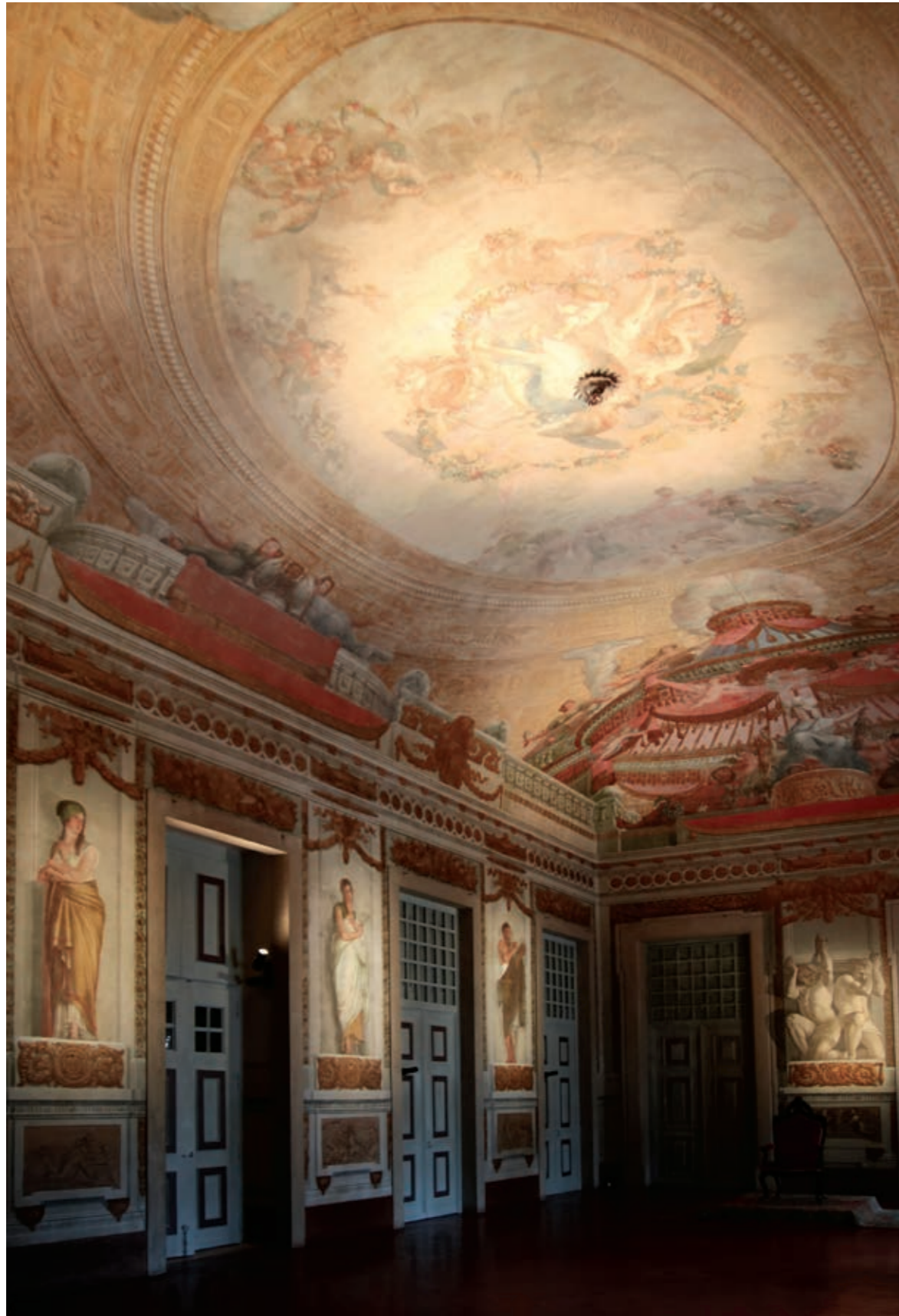
The low-profile luminaires direct the light only where it is strictly necessary.
