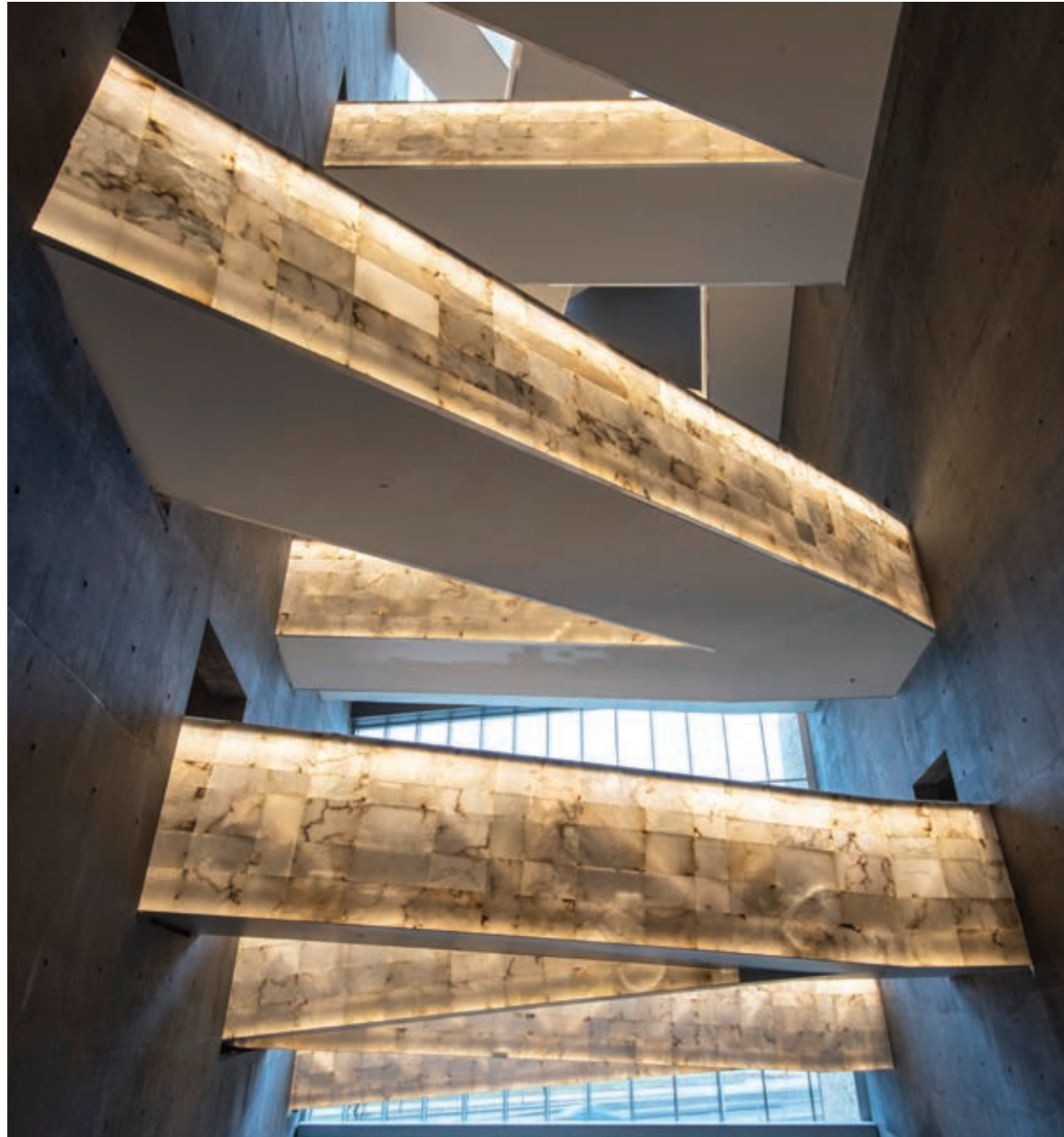
Ultra-compact luminaires are inserted into the alabaster to expose its translucency.
